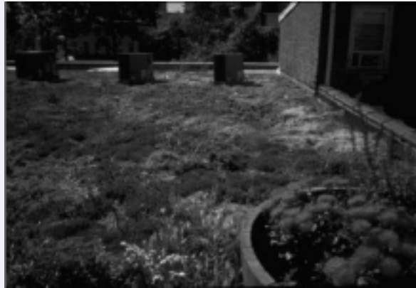
Vegetated roof cover on the Fencing Academy of Philadelphia. Photograph courtesy of EPA
