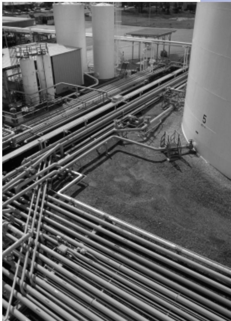
Massive water facilities like this one treat water by removing sludge and scum, aerating the water to eliminate foul odors and tastes caused by decaying organic matter, and killing bacteria through contact with chlorine (which is then neutralized by adding other chemicals). The newly cleaned water is then discharged into a local river or stream. Photograph courtesy of EPA.
