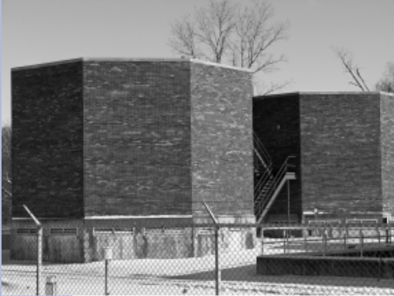
Centralized wastewater treatment facilities like this are the cornerstone of a typical wastewater system.
