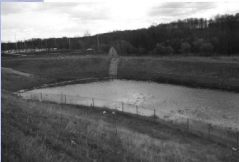
Parking lots like the one in the upper left hand corner of this picture convert rainfall into runoff. The runoff is sometimes impounded in a nearby pond, like this one, where the (often contaminated) water is left to evaporate. Impervious surfaces and their resultant runoff ponds deprive watersheds of the groundwater recharge needed to keep rivers flowing strong. Photograph courtesy of EPA
